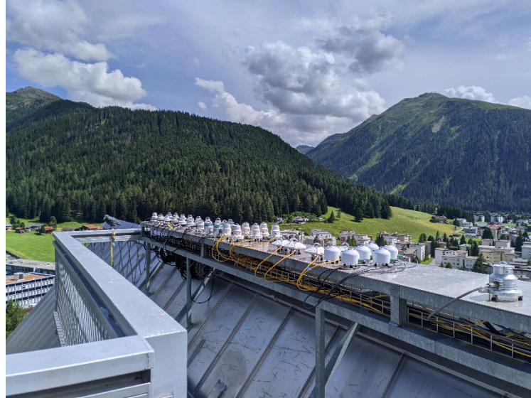
Figure 1. Roof platform of PMOD/WRC.
