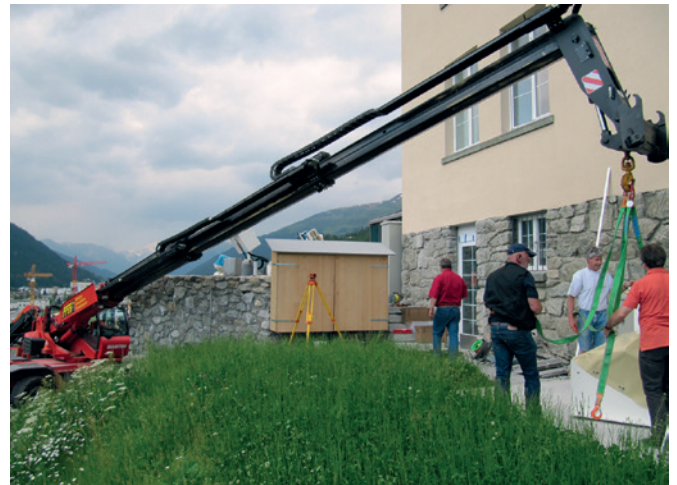
Figure 2. Installation of the Heliostat structure.
