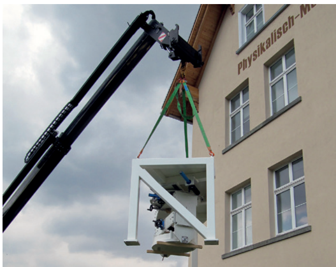
Figure 1. Heliostat structure on the "Manitou" crane in front of the PMOD/WRC building.
