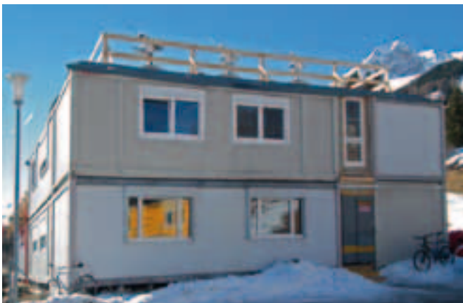
Figure 1. The north side, i.e. the entrance from the car park, of the provisional technical department.
