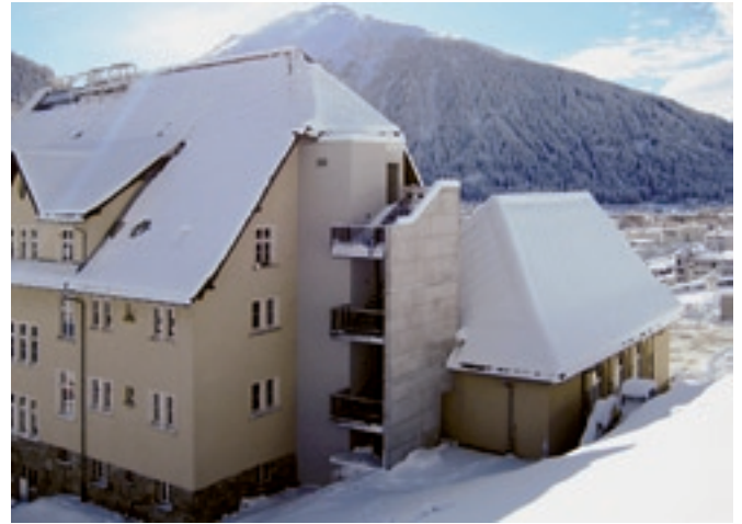
Figure 1. The newly built emergency exit on the west side of the Old Schoolhouse. A new elevator has also been integrated into the structure. Together with an access road behind the mechanical workshop this allows stair-free access of heavy equipment to all floors.
