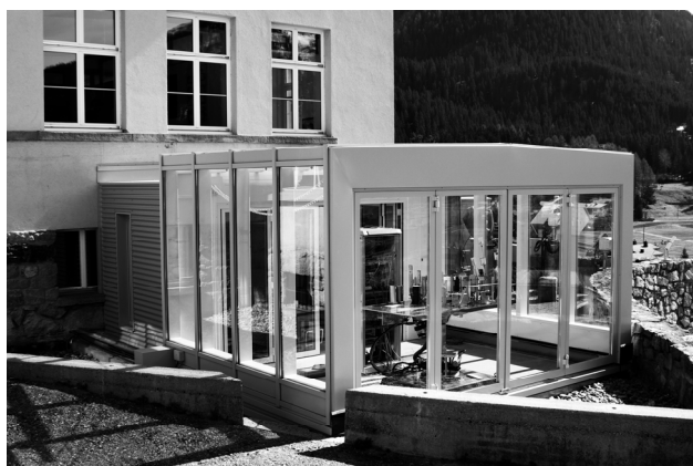
Figure 1 and 2. New glass-building that houses the World Standard Group. Left: Building closed. Right: The front part of the building has been moved back to expose the sun tracker and to enable solar measurements.
